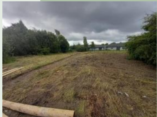
Pond area – work in progress
